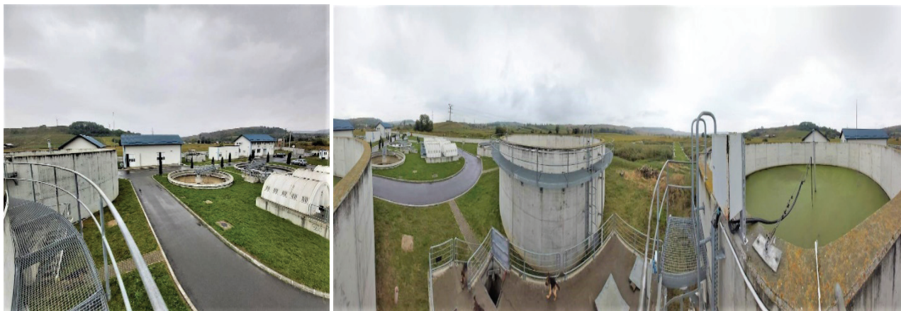
Figure 1. Wastewater treatment plant (original).
